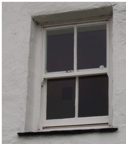
A mid 19 th century sash window with slate sill.
