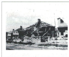
WW2 bomb damage, Holme Lane, Allithwaite 1941
