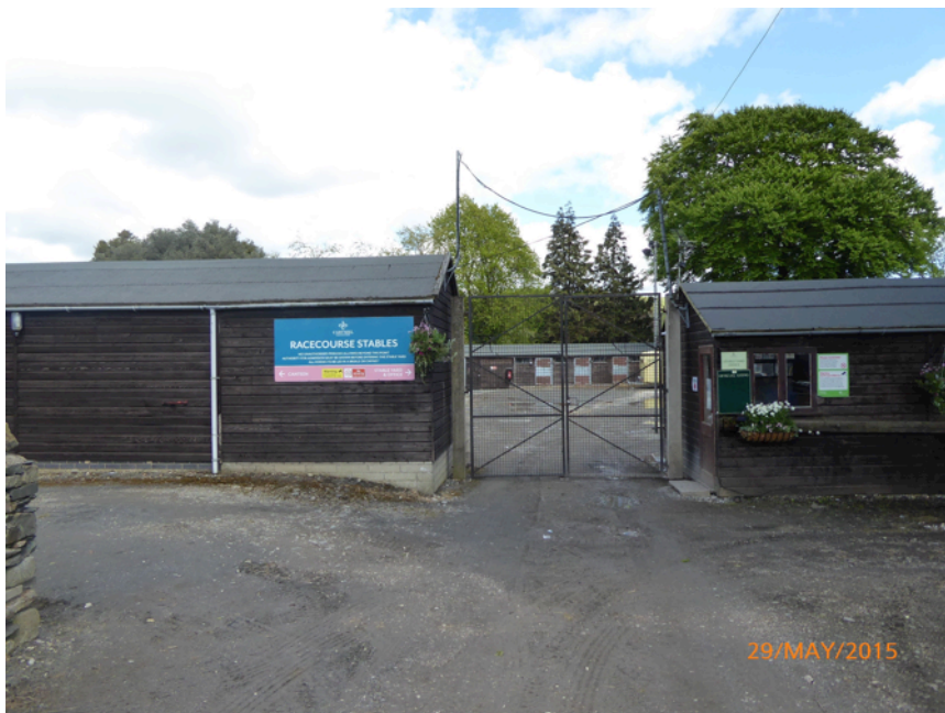
Cartmel Racecourse Loose Boxes.
