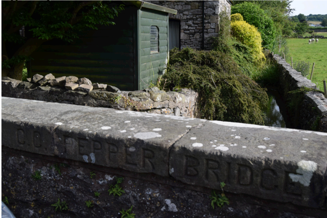
County Council Pepper Bridge
